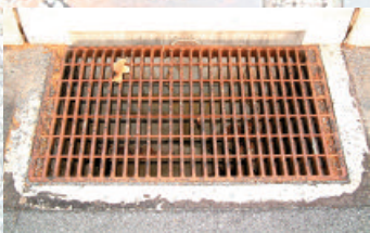
Storm Water Grate
